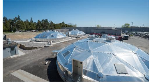
50 feet in diameter and has 16 feet side water depth. During the current upgrades, each clarifier was provided with new dome covers and drive motors were also upgraded to meet electrical code requirements. The domes reduce freezing issues during low flow winter months.
